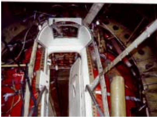
Figure 2-5: DC-9-2 Tail Cone looking forward to bulkhead
