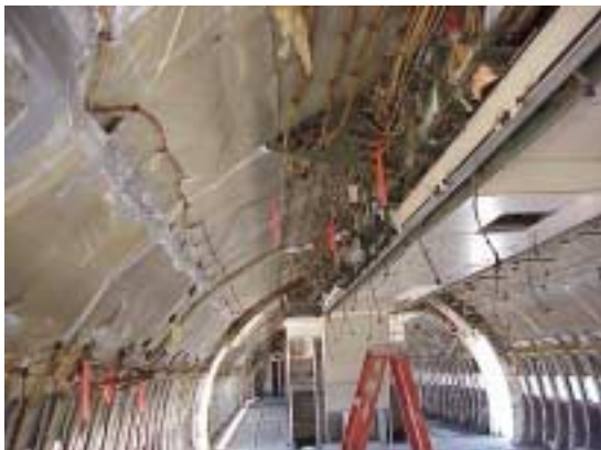
Figure 2-7: L1011 Main Cabin showing PCU cables
