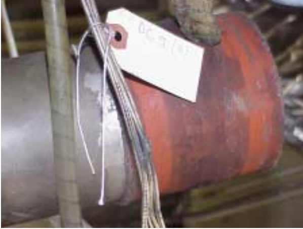
DC-9 Tail Cone Burnt Wires
