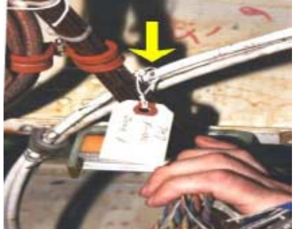
747 Power feeder chaffing
